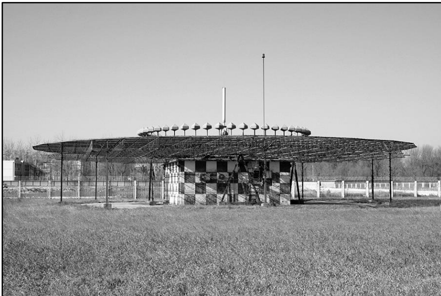
شکل ۹ - VOR/DME ground station
